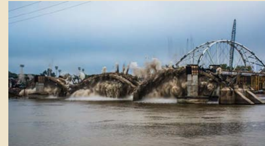
Concrete spandrel arches being demolished in November, 2016. Photo credit: Greg Davis (facebook.com/fastalkr/).
