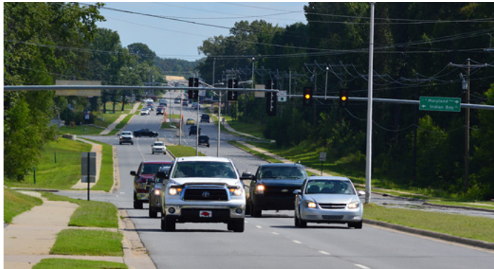
The Regional Arterial Network can take pressure off the freeway system while enhancing suburban mobility.
