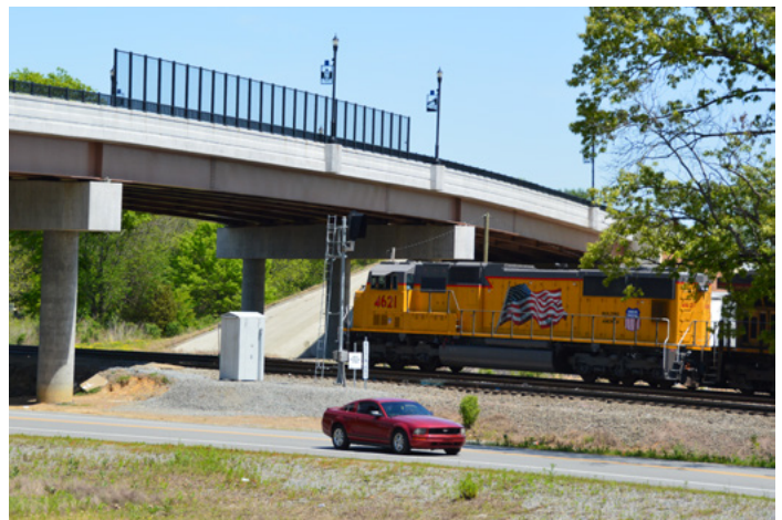
This railgrade separation puts McCain Boulevard above the Union Pacific railroad tracks for mutual benefit.
