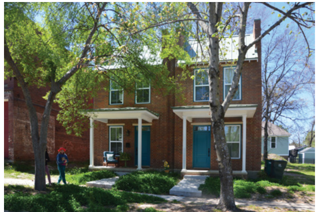
This townhouse-style duplex on Commerce Street, built by Common Ground Development Co., is a winner of the Richard Butler Award of Merit for Infill Development from the Quapaw Quarter Association.
