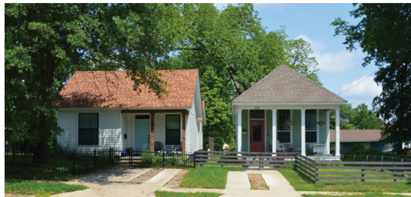
These new single-family houses on East Charles Bussey are examples of a side courtyard style (left) and shotgun style (right).
