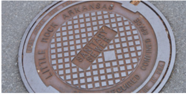
A sewer manhole cover.
