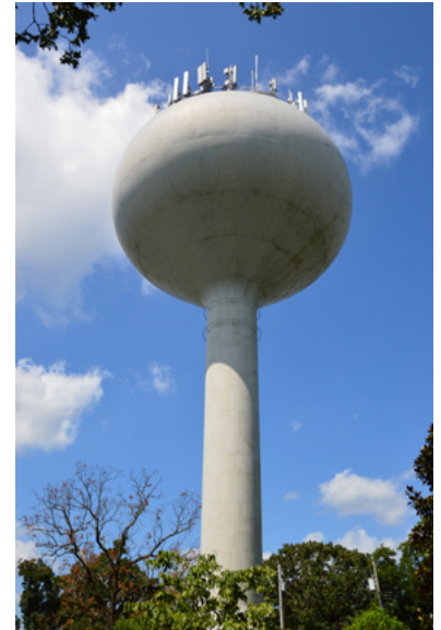
Examples of antennas attached to existing structures.
