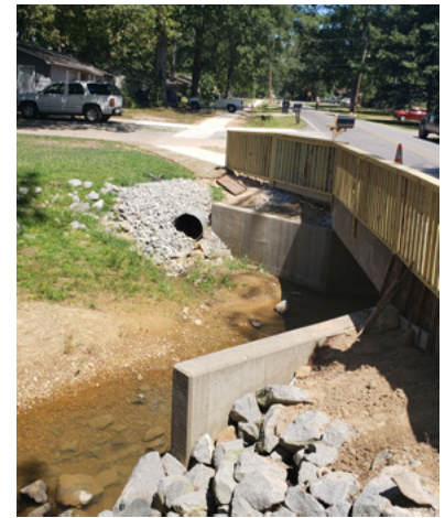
Box culvert with sidewalk.
