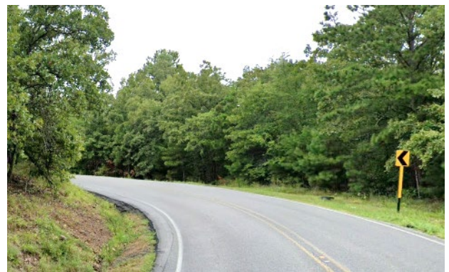
Figure 27: The superelevation on northbound Batesville Pike is sloped towards the outside of the curve at the first left curve north of Greer Road.
