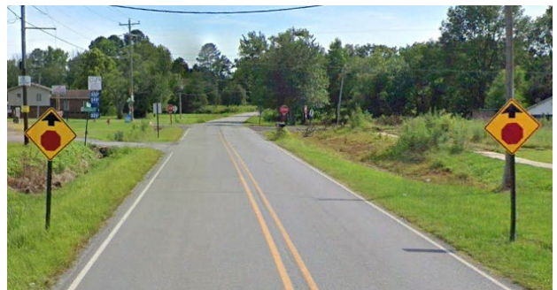
Figure 7: Stop ahead warning signs are double posted for the southbound approach of Batesville Pike to Jacksonville Conway and signs are located approximately 180-feet in advance of the intersection.
