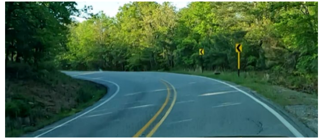
Figure 13: Chevron signs do not continue through the entire curve for northbound vehicles on Batesville Pike at the 'S' curve between Angel Lane and Greer Road.
