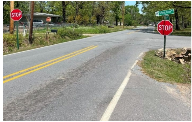
Figure 29: Bottom of existing stop sign at the northbound approach of Batesville Pike to Kellogg Acres Road is posted at 3-feet and 4-inches above the surface of the pavement.
