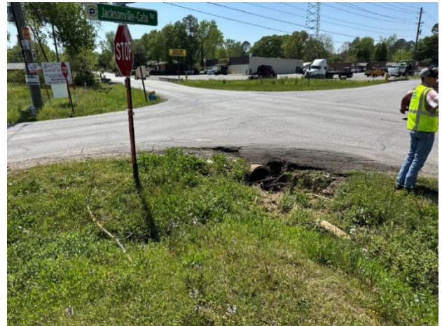
Figure 28: Intersection of Batesville Pike and Jacksonville Cato Road with a drainage ditch close to the edge of pavement at the northeast corner.
