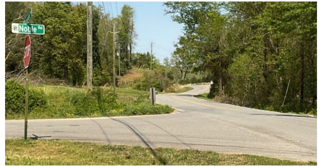
Figure 9: Intersection within curve near where no warning signs exist in advance of the intersection.
