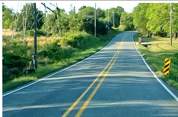
Figure 5: Object markers only on the right side of a culvert in both directions on Batesville Pike between Northview Road and Angel Lane.
