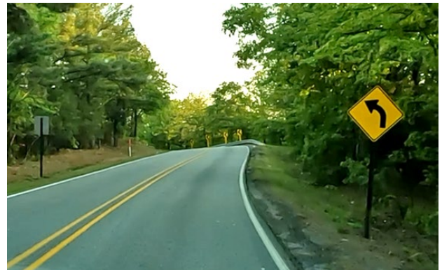
Figure 26: Left curve warning sign on southbound Batesville Pike just south of Angel Lane, however the road is curving right.
