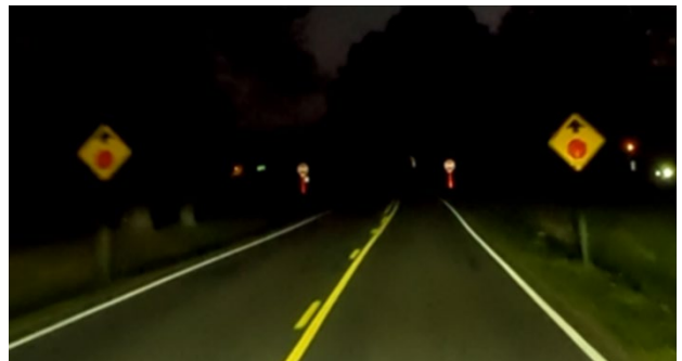
Figure 8: Double posted stop ahead warning signs and stop signs with red reflective tape on the sign posts located at the southbound approach of Batesville Pike to Republican Road.
