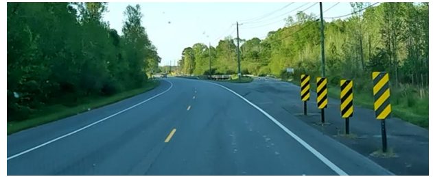
Figure 18: Object markers posted along the northbound approach of Batesville Pike to the decommissioned bridge alignment, south of Frenchman Mountain Road.
