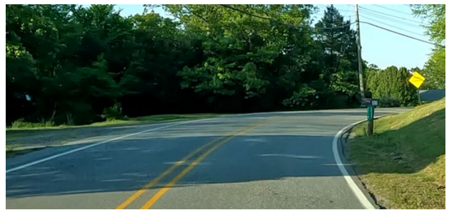
Figure 24: Chevron signs do not exist along the less severe curve at the northbound approach to a 90-degree curve just south of Northview Road.
