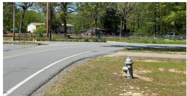
Figure 33: Kellogg Acres Road centerline stripe is curved to guide westbound vehicles approaching Batesville Pike to turn right.
