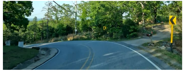
Figure 12: Chevron signs do not continue through the entire curve for vehicles on northbound Batesville Pike at the 90-degree curve near Northview Road.
