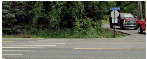
Figure 31: Existing skewed crosswalk across the north leg of the intersection of Pine Street and Main Street leads pedestrians to a ditch at the northeast corner.
