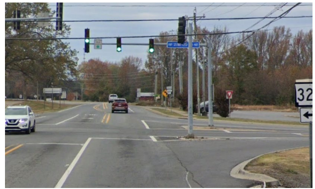
Figure 42: Existing traffic signal pole for signals serving the westbound approach of Bill Foster Memorial Highway blocks the street name sign on the mast arm for the southbound approach of Pine Street.
