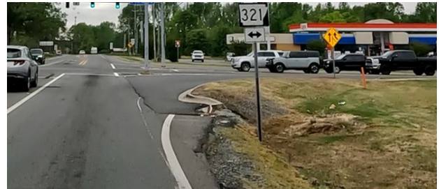
Figure 41: Existing Pine Street southbound right-turn channelized lane curb does not align with edge line to protect approaching turning vehicles from the ditch.
