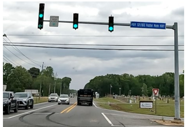
Figure 38: Existing left-turn signal head with a green ball and arrow and sign for left-turn vehicles to yield on green ball for northbound vehicles on Pine Street at Bill Foster Memorial Highway.
