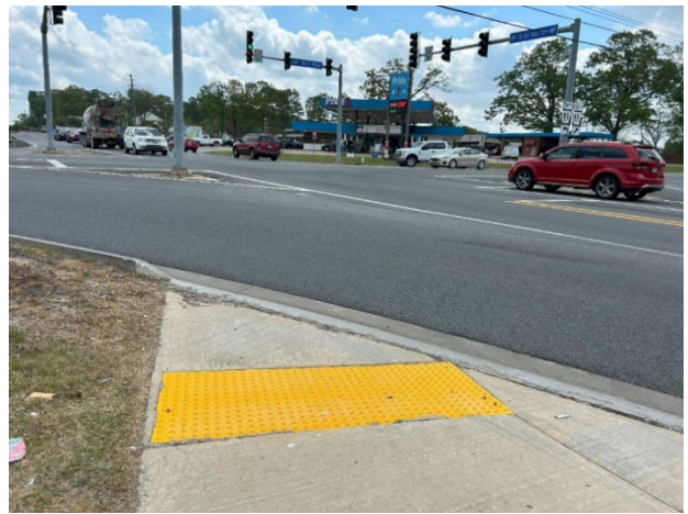
Figure 43: Existing ramp at the northwest corner does not lead to a crosswalk or connect to any other pedestrian infrastructure.
