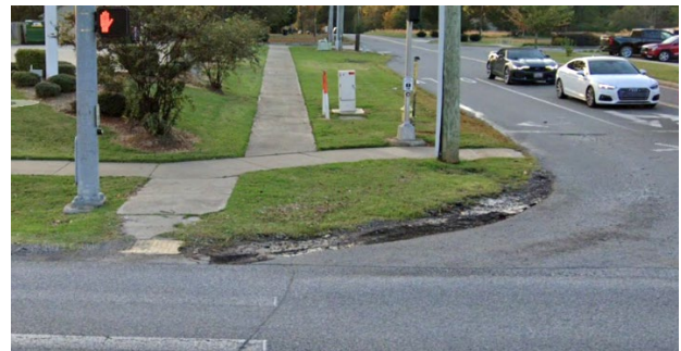
Figure 34: Southwest corner of Pine Street and Campground Road where vehicles have cut the corner and have worn down the pedestrian ramp.
