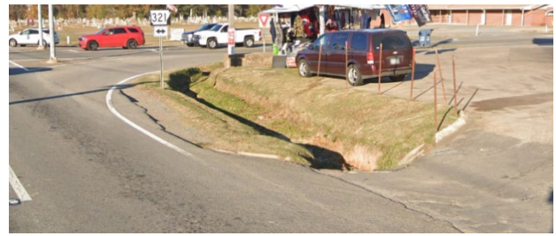
Figure 40: Existing pavement drop-off at the southeast corner of Pine Street and Bill Foster Memorial Highway. (Photo provided by Google Street View April 2025)
