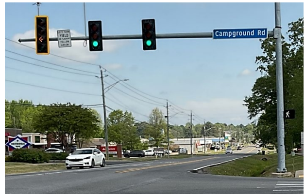
Figure 8: Existing traffic signal at Pine Street and Campground Road with a retroreflective backplate installed only on the northbound left-turn signal head.
