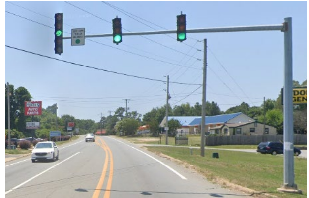
Figure 13: Left-turn signal head on southbound Arch Street Pike with a green ball and sign for left-turn vehicles to yield on green.
