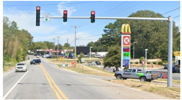
Figure 12: Traffic signal heads at Pratt Road and Arch Street Pike with no backplates.
