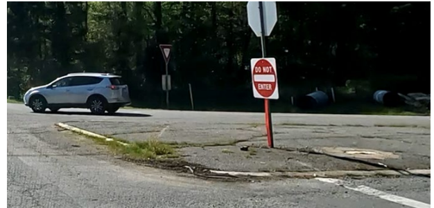
Figure 21: Corners of raised concrete islands are in disrepair and vegetation appears to be causing additional damage.
