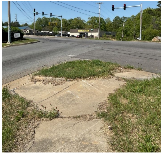
Figure 14: Existing sidewalk on the raised concrete channelization island for right-turns from westbound Pratt Road to northbound Arch Street Pike.
