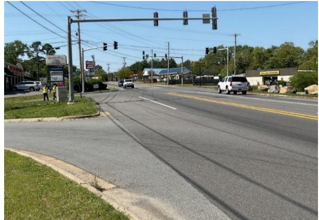
Figure 11: Extra pavement exists between the northbound receiving lane on Arch Street Pike and the raised westbound right-turn channelization median for Pratt Road.
