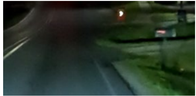
Figure 7: Mailbox near McDonald's driveway does not have a reflective object marker for westbound vehicles.
