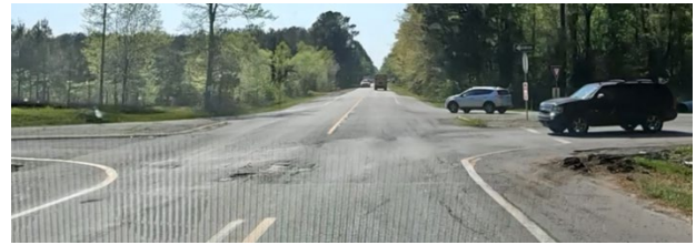
Figure 20: Raised concrete islands are nearly flush with the pavement.
