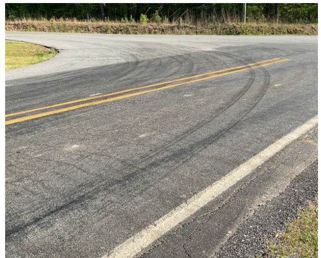
Figure 18: Tire marks from large vehicles on westbound Pratt Road turning right onto northbound Ironton Road but swinging wide and entering the southbound Ironton Road lane.
