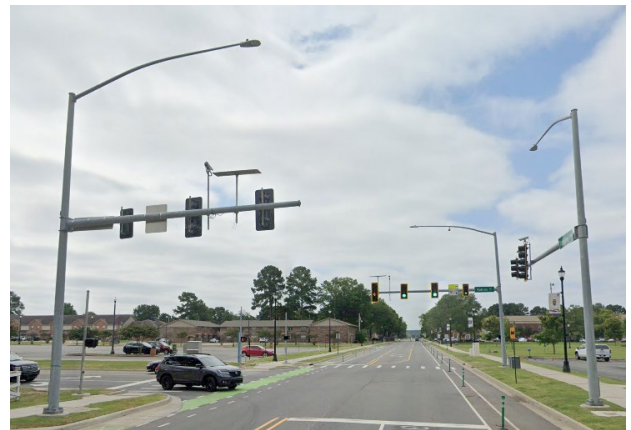
Figure 20: Existing intersection lighting on traffic signal poles at the South Donaghey Avenue and Robins Street intersection.
