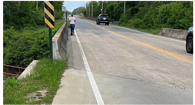
Figure 36: Pedestrian crossing Stone Dam Creek bridge in the narrow shoulder.
