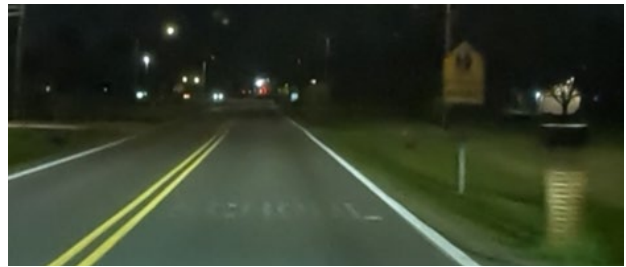
Figure 5: Northbound approach to the school zone warning sign at Favre Lane is not retroreflective and the SCHOOL pavement marking is faded.
