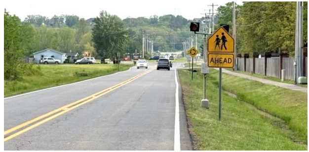
Figure 42: The school zone ahead warning sign on southbound South Donaghey Avenue blocks the view of the flashing beacons for southbound vehicles approaching Favre Lane.
