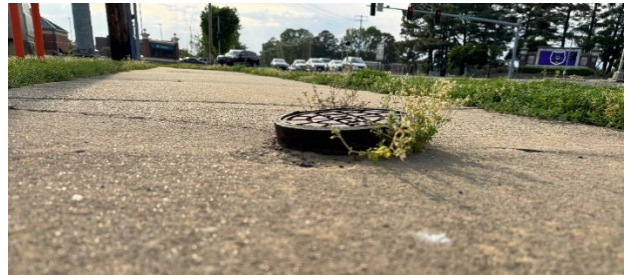
Figure 24: Water line access cover raised 1.75" above sidewalk surface near the southeast corner of South Donaghey Avenue and Dave Ward Drive.
