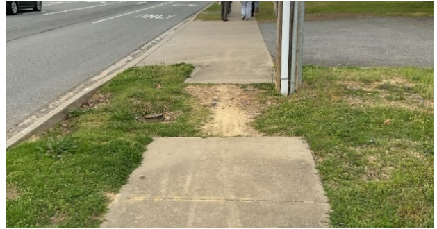
Figure 23: Section of sidewalk is missing on the east side of South Donaghey Avenue south of Dave Ward Drive.
