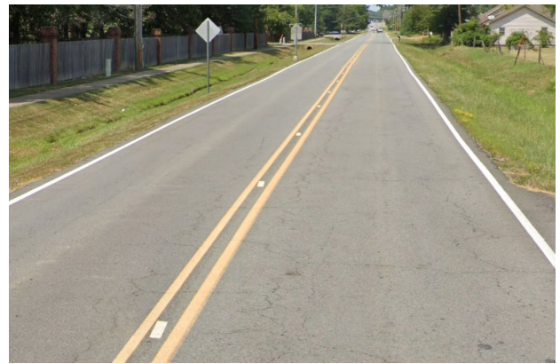
Figure 35: White dashed pavement marking along the centerline striping of South Donaghey Avenue near the northbound approach to Attwood Drive.
