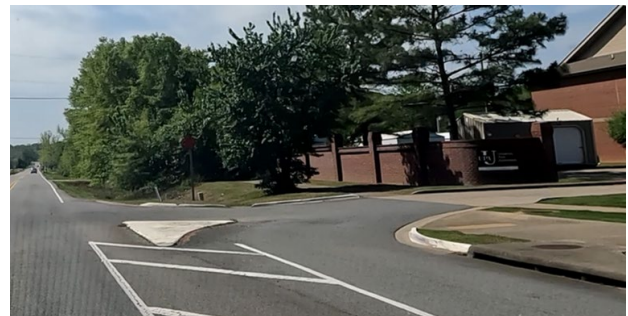
Figure 33: Raised concrete channelization island and pavement markings for the southbound right-turn lane along South Donaghey Avenue for the University Park Apartments Driveway.
