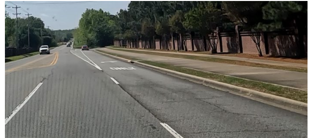
Figure 32: White dashed lane lines leading up to the southbound right-turn lane for the University Park Apartments Driveway.
