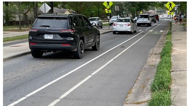
Figure 17: Several delineators for the bike lane are missing along the west side of South Donaghey Avenue near the RRFB closest to Bruce Street.
