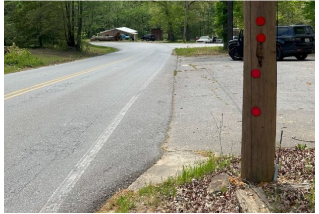
Figure 29: Utility pole that appears new with reflective object markers at the southbound approach of Vimy Ridge Road to Barth Road.
