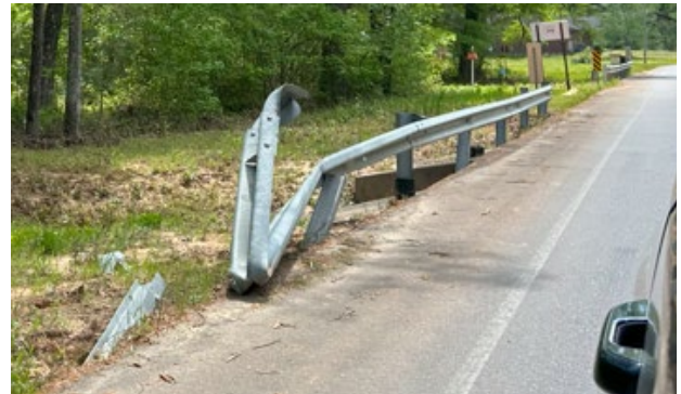
Figure 35: Guardrail is damaged along the east side of Vimy Ridge Road.
