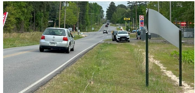
Figure 14: The existing lane assignment sign for northbound Vimy Ridge Road was facing the wrong direction due to damage from a recent storm.
