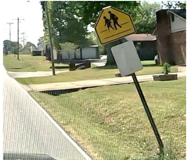
Figure 19: Existing school crossing warning sign and faded sign underneath at the southbound approach to Packer Drive.
