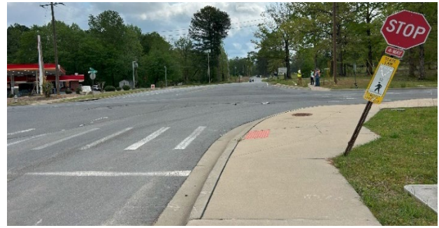
Figure 12: A stop sign for the eastbound approach was tilted away from the intersection.
