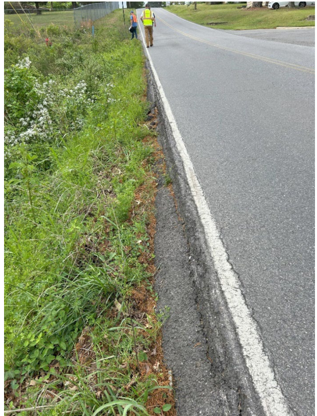
Figure 10: Steep drop off from the surface of pavement to the ditch along the east side of Vimy Ridge Road south of County Line Road.
