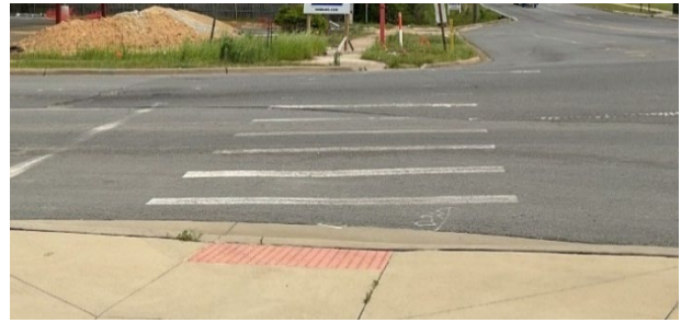
Figure 11: Faded crosswalk markings for crossing the west leg of the intersection and diagonal ramp at the northwest corner.
