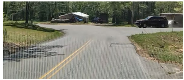
Figure 25: Southbound approach to Barth Road has no curve or intersection warning signage or chevrons.
