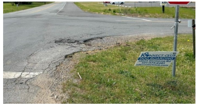
Figure 41: Degraded pavement at the northwest corner of the intersection of Vimy Ridge Road and Germania Road.
