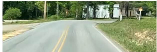
Figure 26: Northbound approach to Barth Road has no curve or intersection warning signage or chevrons.
