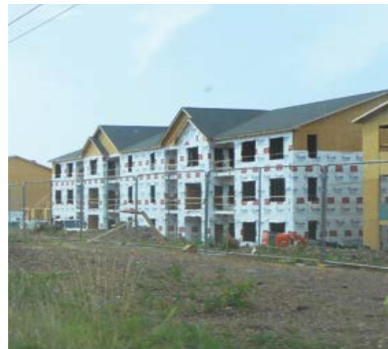
A slight reduction in travel times from the I-430/630 interchange rebuild may convey a development boost to western Little Rock. The McKenzie Park apartments, seen here under construction, will add 168 units along Kanis Rd.
