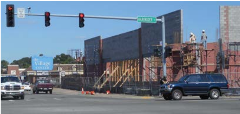
This CVS pharmacy under construction along Oak Street, just east of downtown Conway, is built up to the street front with parking in back. Over time, street-front projects like this should transform the western portion of Oak St. into a more pedestrian-friendly urban format.
