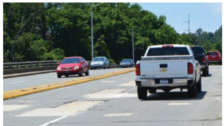
This bridge just west of downtown on Cantrell Road exemplifies the deferred-maintenance problem.
