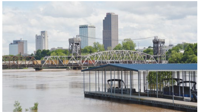
The Rockwater Marina rode out the high water in 2019 without damage. Rockwater residents enjoy views of the Arkansas River and downtown Little Rock, as well as easy access to Argenta in North Little Rock
