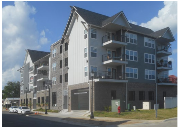
The J Lofts Apartments blend into the urban fabric in Conway's revitalizing downtown.
