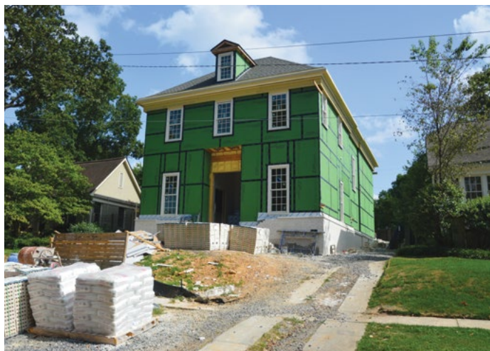
Tear-downs are followed by larger rebuilds in Little Rock's Heights neighborhood.
