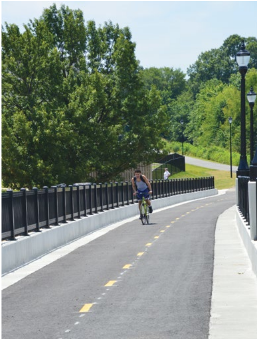
A new bridge gives those living south of Dave Ward Drive direct access to the UCA campus.
