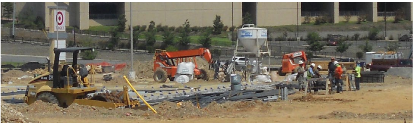
Construction of the Park Avenue Center continues a mid-town retail comeback in Little Rock.
