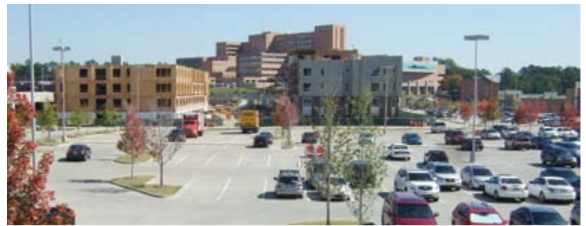
These images from 2009 (above) and 2012 (below) convey the gradual transformation of the old University Mall site into the mixed-use Park Avenue Center.
