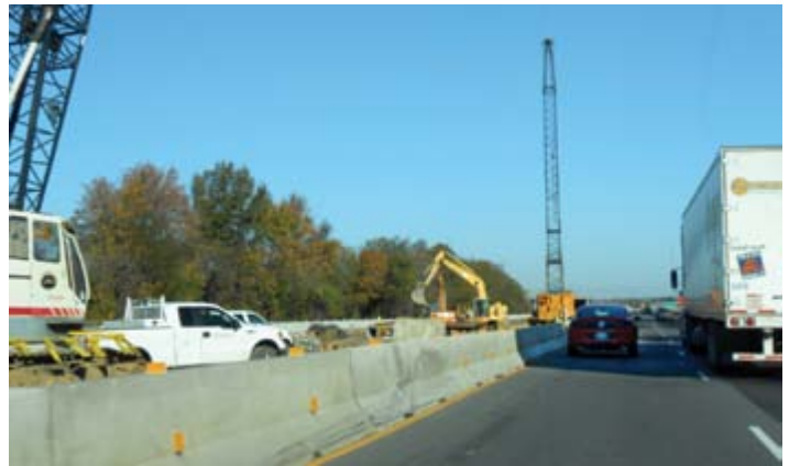
Widening work now underway will yield six travel lanes on I-40 between Conway and North Little Rock.
