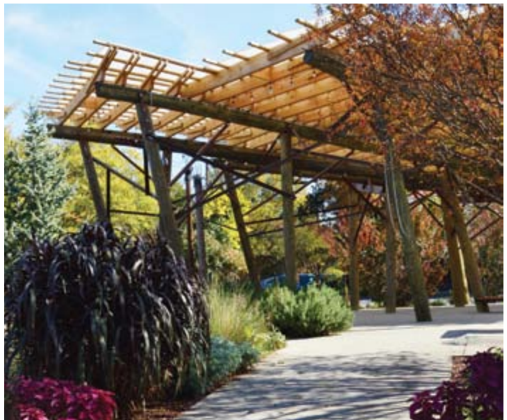
Ms. Davis collaborated with area architects and students from the University of Arkansas at Little Rock, to build the Bernice Garden pavilion. It is made from recycled and reclaimed materials and features LED lighting and a cistern to collect rainwater for the garden.
