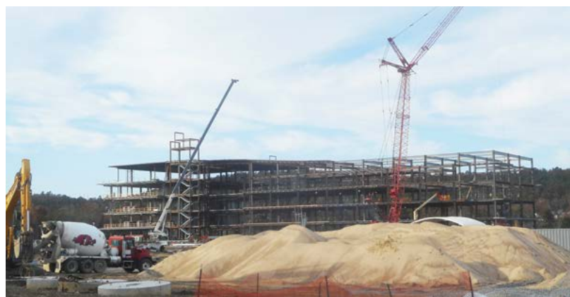
Tipping the scales at nearly $100 million, the new Bank of the Ozarks headquarters on Cantrell Road in western Little Rock demonstrates the local finance industry's competitive strength.
