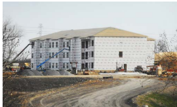
This is the first of several new multi-family structures along North Hills Boulevard in North Little Rock. When complete, the new complex could contain up to 900 new units.
