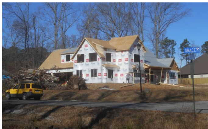
Upscale home under construction in southeastern Bryant.
