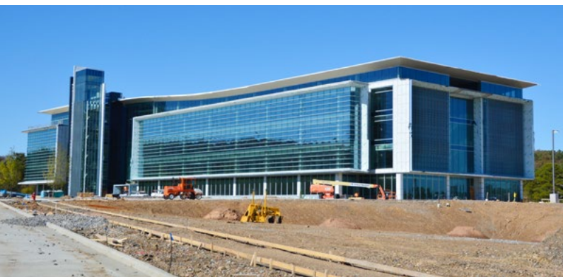
The new headquarters for Bank OZK. Now the region's largest bank, it also has a major presence in commercial construction investments in New York and California.
