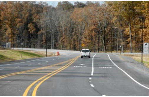
White Oak Crossing interchange.
