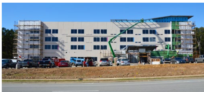
The $13.7 million Aloft Hotel (above) and a 300-unit apartment complex (below) mark a continuing trend of investment near the Promenade at Chenal.
