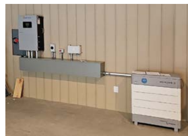
With a compact battery like this, residential users get a backup generator for emergencies when the grid goes down.
