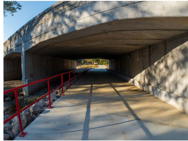
Salem Road Bridge and Pedestrian Underpass in Conway. The project replaced the existing Salem Rd Bridge over Tucker Creek with a longer and wider bridge that accommodates an underpass of Kinley Trail below the roadway. Multi-use paths and sidewalks were added along Salem Rd to provide additional connectivity to the trail system. Photo credit: City of Conway, Arkansas.
