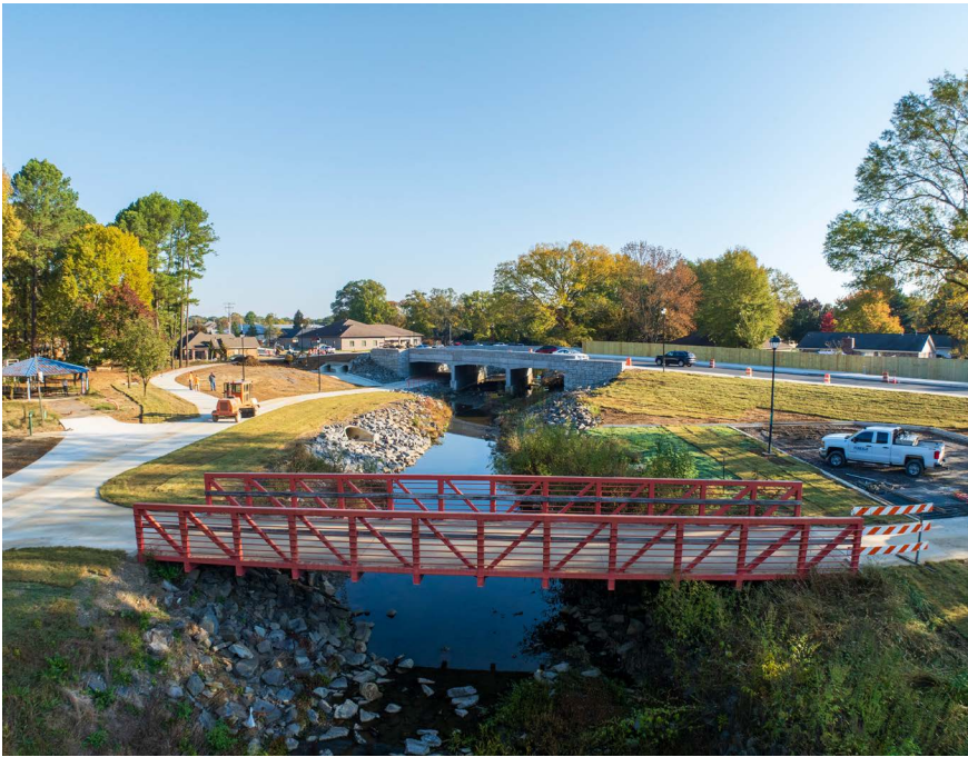
Salem Road Bridge and Pedestrian Underpass in Conway. The project replaced the existing Salem Rd Bridge over Tucker Creek with a longer and wider bridge that accommodates an underpass of Kinley Trail below the roadway. Multi-use paths and sidewalks were added along Salem Rd to provide additional connectivity to the trail system. Photo credit: City of Conway, Arkansas.
