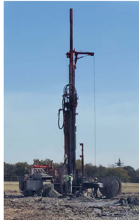
Metroplan's EPA CPRG grant funded the construction of 170 geothermal wells, which provide the foundation for the Clinton National Airport's new Central Utility Plant. Using geothermal to heat and cool the terminal will reduce the airport's electricity consumption and nearly eliminate its use of natural gas.
